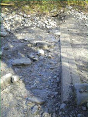
Surface repaired by Denbighshire County Council in 2008 now eroded into step.
